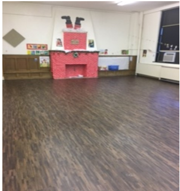
After, new vinyl plank flooring
